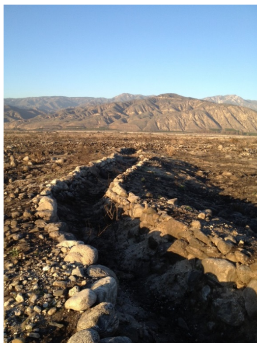
Judson and Brown Ditch, San Bernardino County
