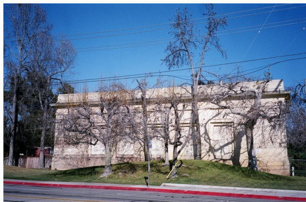
San Diego Gas & Electric San Juan Capistrano Substation, San Juan Capistrano, Orange County
