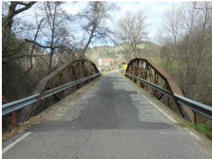
Calaveritas Creek Bridge, Calaveras County
