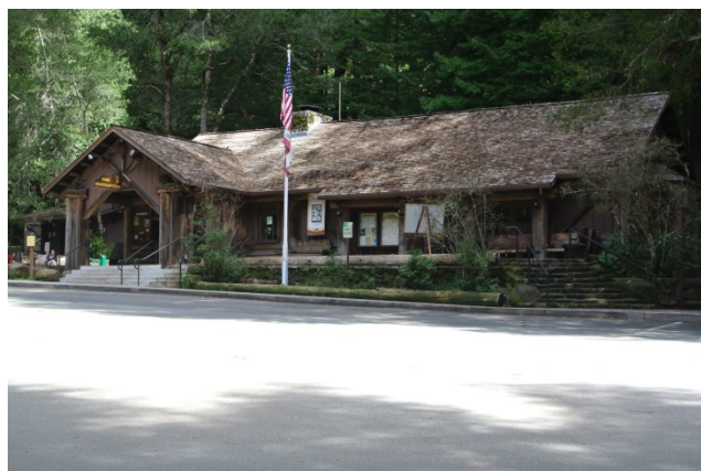
Headquarters Administration Building, Santa Cruz County
