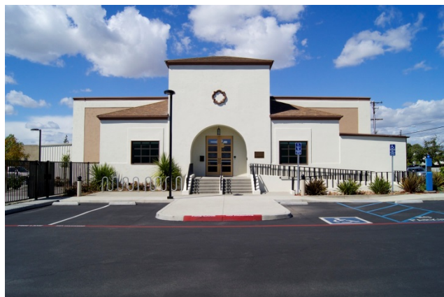
Cypress Street Schoolhouse, Orange County
