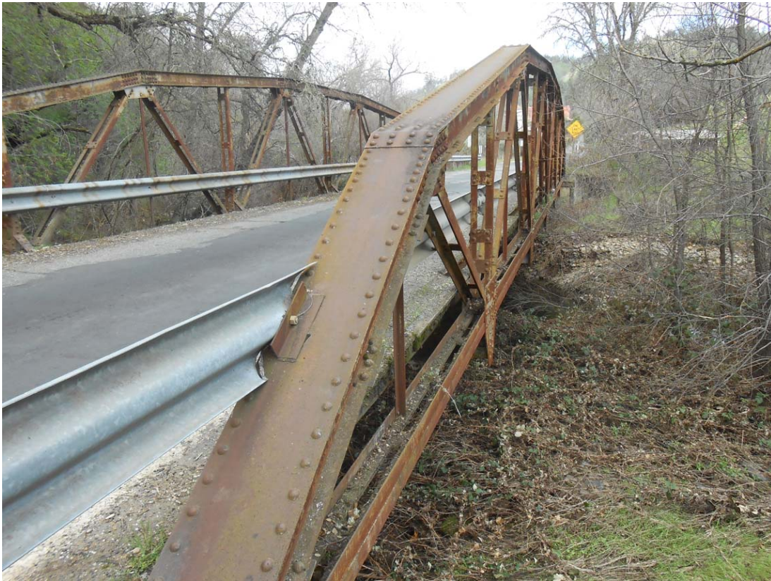
Calaveritas Creek Bridge, Calaveras County
